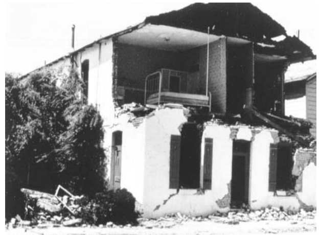
Figure 21 - The plaster-covered brick walls of this building collapsed during a recent earthquake.
