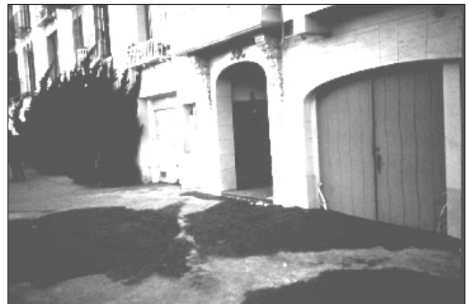
Figure 36 - Loma Prieta Earthquake, October 17, 1989. Lateral spreading, liquefaction and sand boils caused extensive damage in the Marina District of San Francisco, about 60 miles away from the epicenter.
