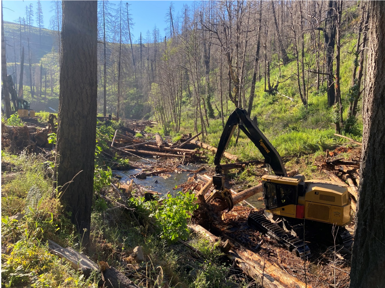
Figure 1-2: Gate Creek Large Wood Placement
