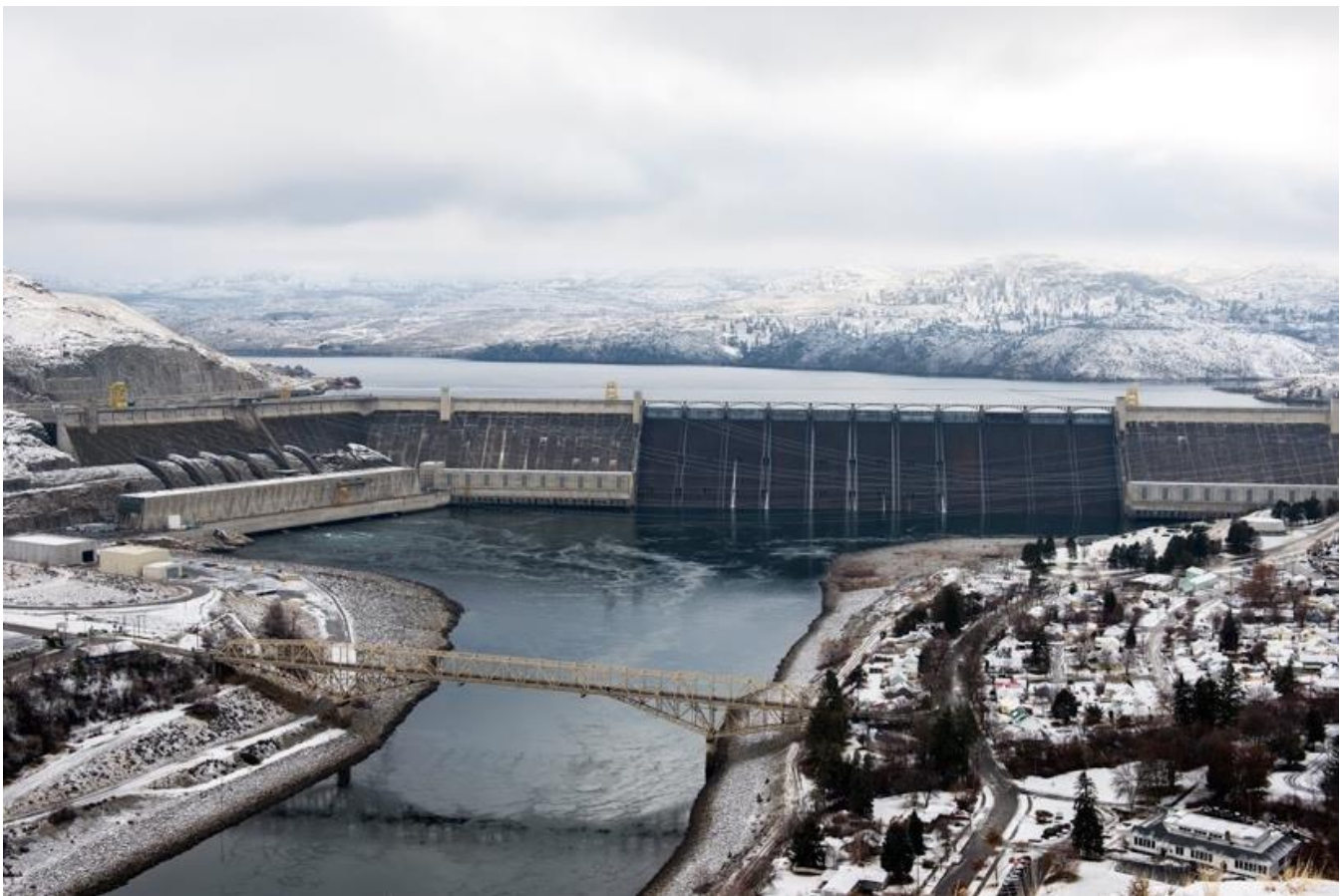
Grand Coulee Dam in the winter. Courtesy of the Bureau of Reclamation.
