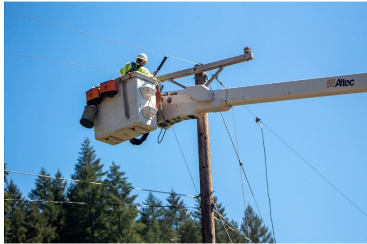
2022 single-phase reconfiguration work
