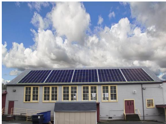
Improvised view of final installation
