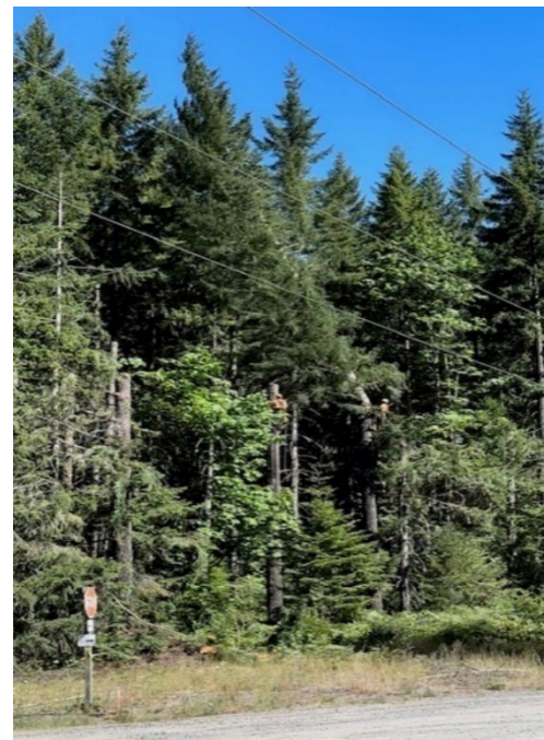
EWEB Contractors Topping Trees
