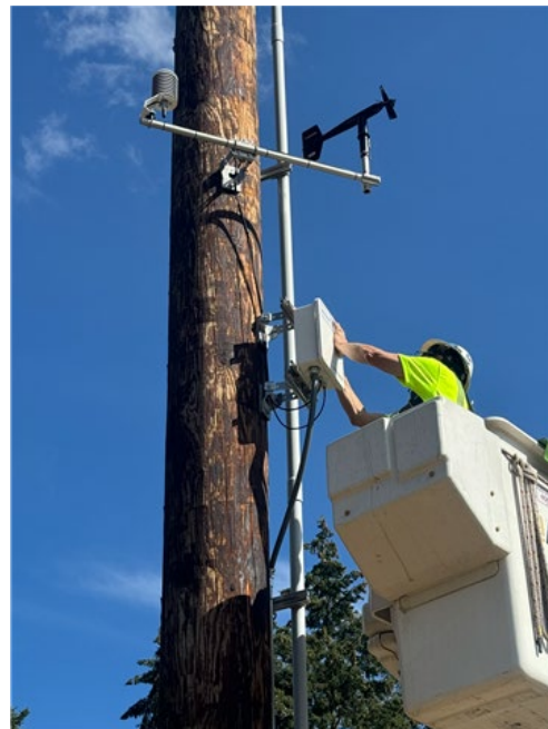
Weather station install on EWEB pole
