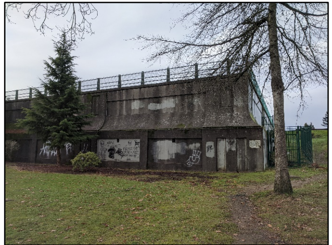
Figure 3.3-6. College Hill Reservoir 607, east face, north end; view southwest.
