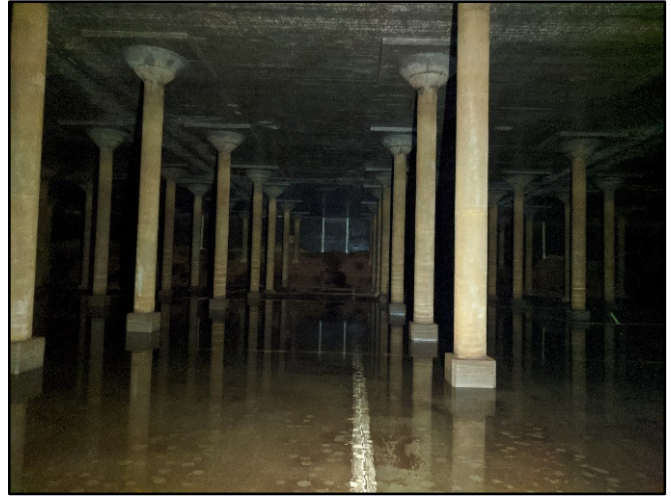
Figure 3.3-10. North reservoir area, view north.
