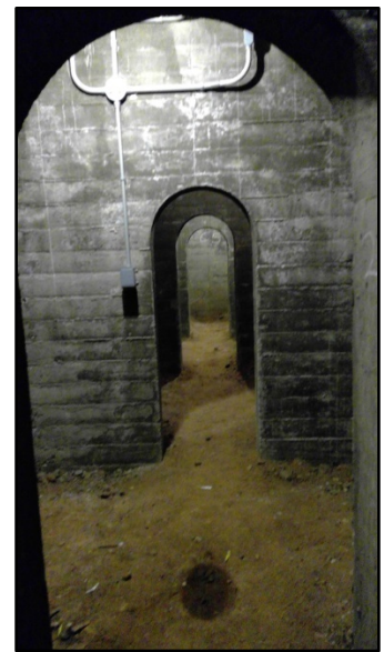
Figure 3.3-12. Catacombs beneath College Hill Reservoir 607; view west.
