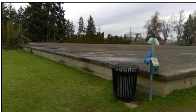
Figure 3.1-1. College Hill Reservoir 603; view northeast.
