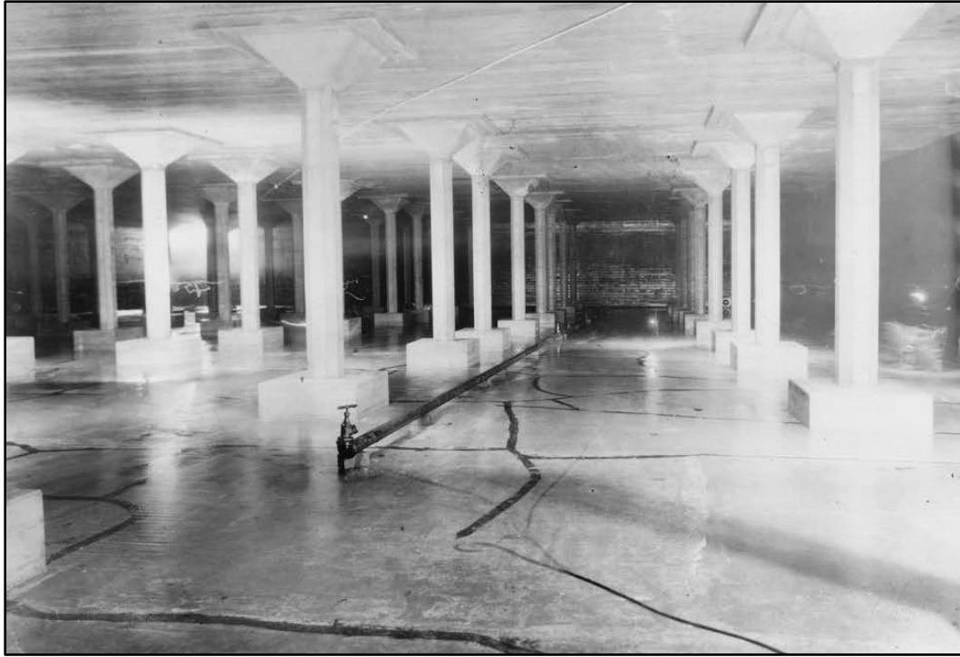
Figure 3.1-8. Interior of College Hill Reservoir 603 after completion of cover, December 26, 1933. Photo by Dot Dotson. Image 1246, courtesy of EWEB.
