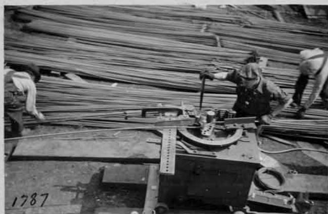
No.1-Improved method of oiling capitol forms. No.2-Dist. method for roof concrete pour. No.3-General view and runway system on roof concrete pour. No.4-Rodding a section of roof slab. No.5-Closeup showing consistancy of concrete. No.6-Application of Broom Finish. No.7-Straightening and rebending wrongly bent reinforcing steel.
