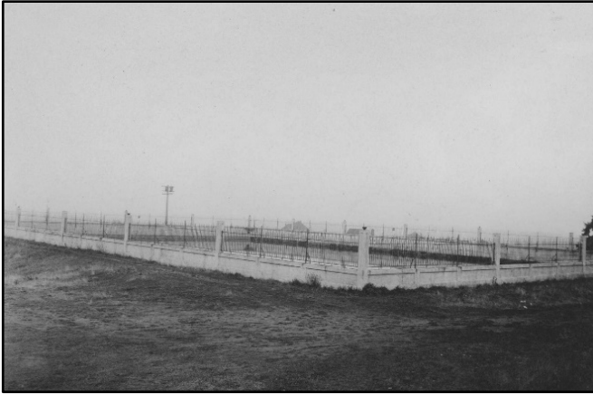
Figure 3.1-5. College Hill Reservoir 603, approximately July 1931; view southwest. Image courtesy of EWEB.
