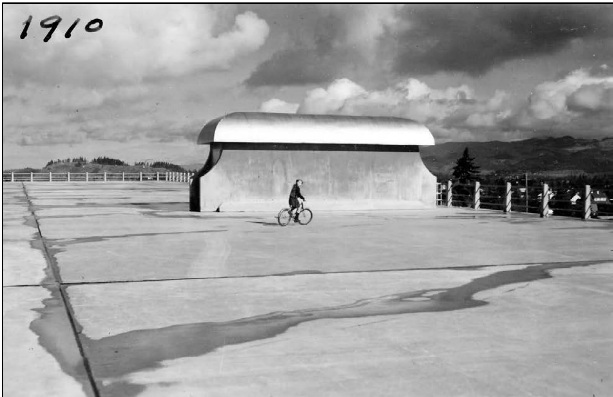
Figure 2-1. College Hill Reservoir No. 2, February 11, 1940, looking north at entrance house structure. EWEB Image No. 1910, courtesy of EWEB.
