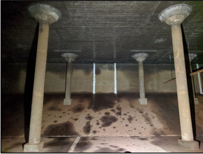
Figure 3.3-9. North reservoir area, with detail of columns and roofs, view south.
