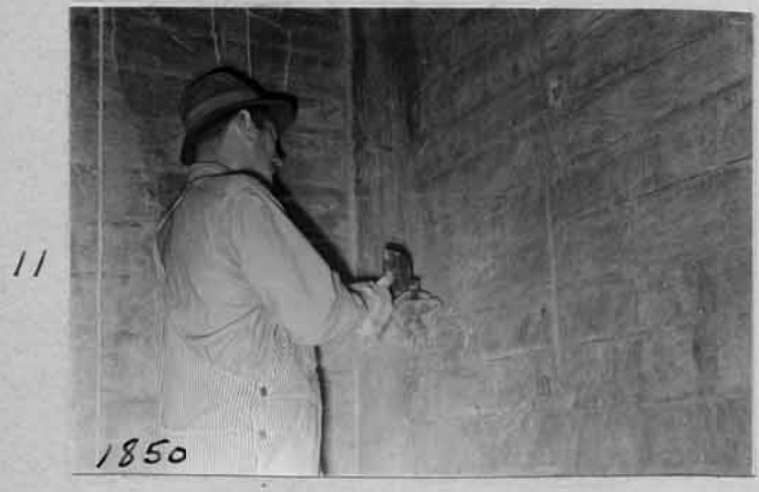
No.7- From Lawrence St. to 23rd. St. prior to grading. No.8- Entrance chamber during construction. No.9- Stripping roof forms.(South Basin) No.10- Chipping and plastering end of closing sections. No.11-Chipping and patching wall(North Basin) (In this particular instance a 2x2" form spreader was left in the wall. No.12-Pouring tar in slope slab expansion joints.
