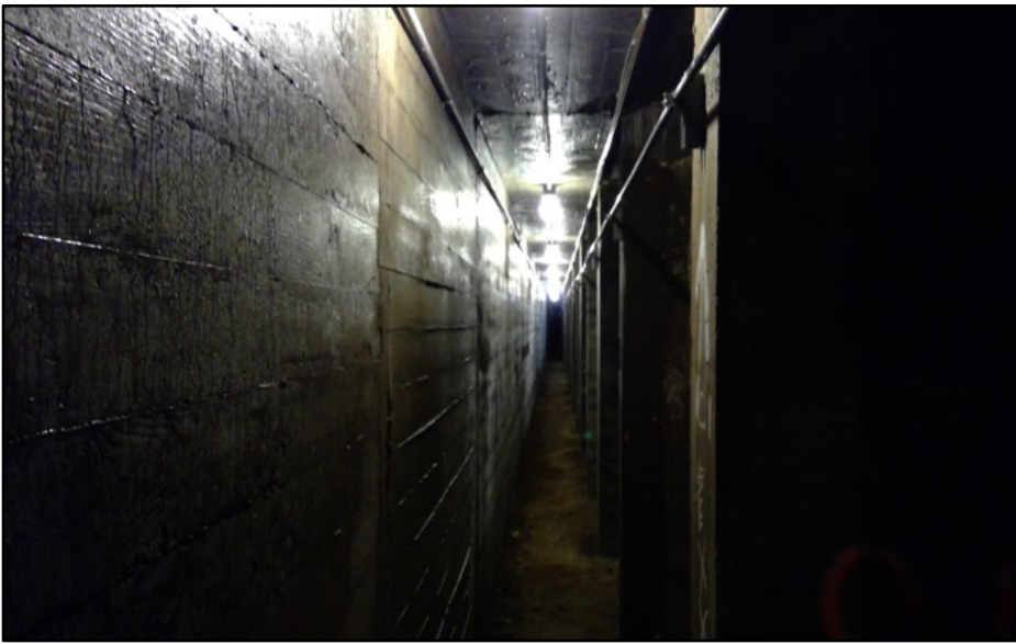
Figure 3.3-11. Catacombs beneath College Hill Reservoir 607; view south.
