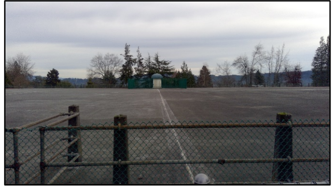
Figure 3.3-2. College Hill Reservoir 607 roof and entrance structure; view east.
