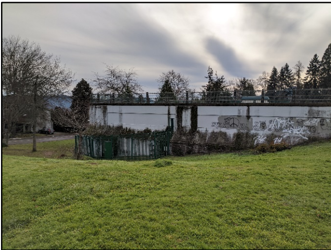
Figure 3.3-5. College Hill Reservoir 607, north face, east end; view southeast.
