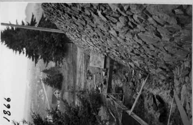
Nos.1 to 8 Inclusive . All pictures of hand placed rock by pump house.
