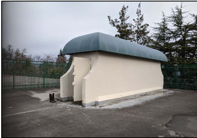
Figure 3.3-7. Entrance structure atop College Hill Reservoir 607; view northeast.
