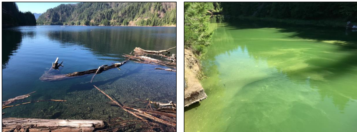
Figure 3-3: Cougar Reservoir (left) and Blue River Reservoir (right) on 7/13/2020
