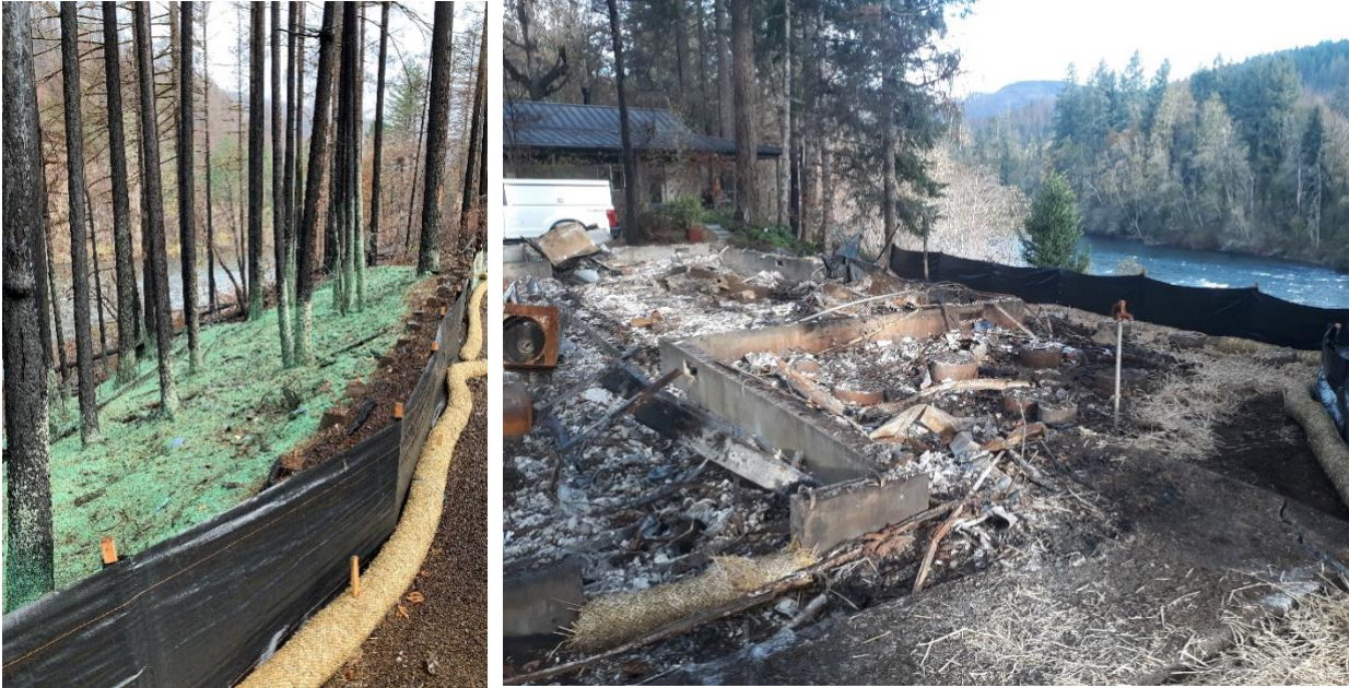
Figure 7-1: Hydroseeding, Wattles, and Silt Fences
