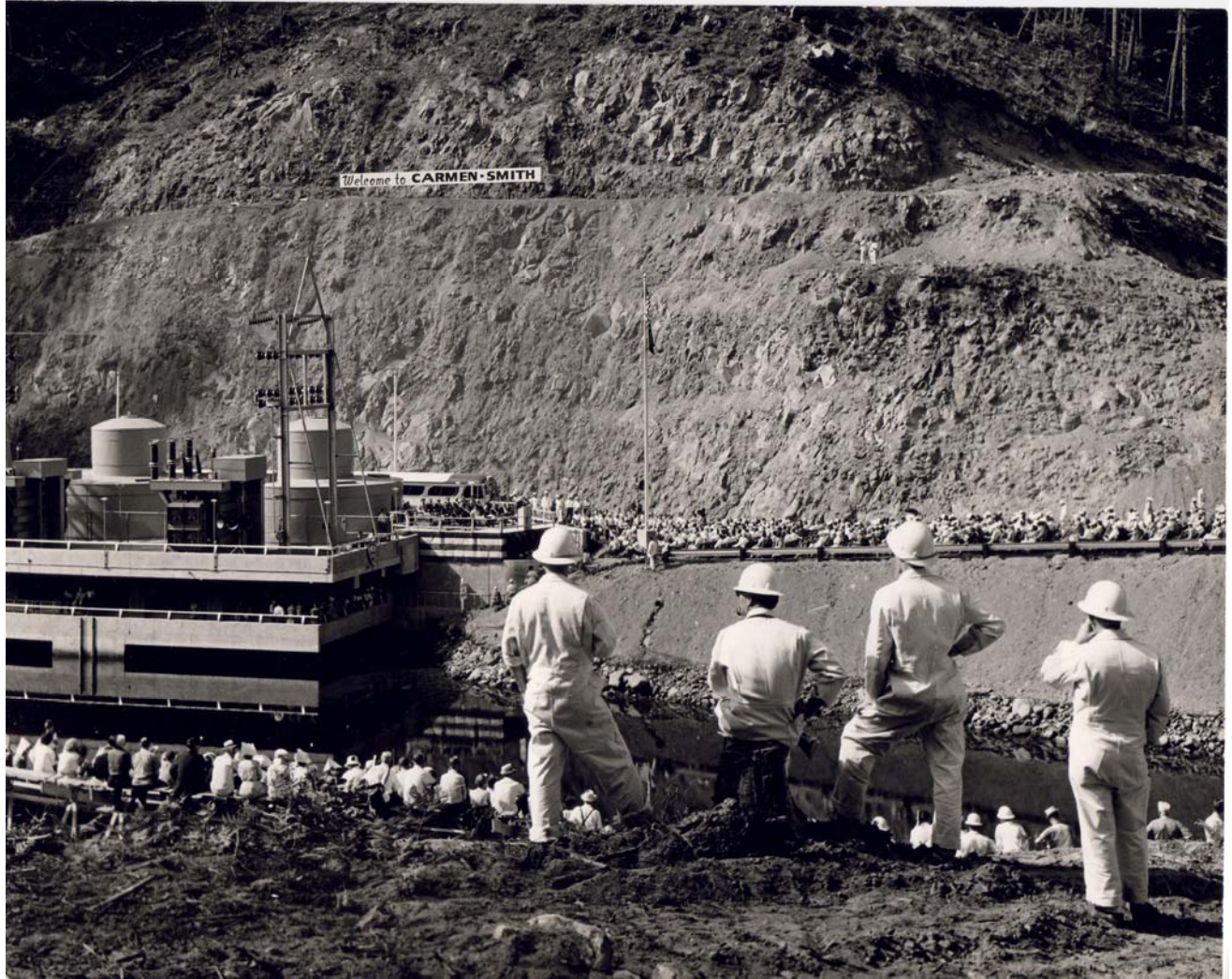
Carmen Powerhouse Dedication, September 1963
