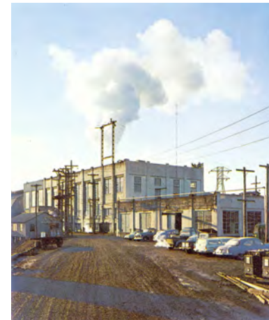
Figure 2-128 Plant in 1960 before roadway was paved
