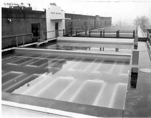
Figure 4-94 Looking north from south #3 filter - 1963
