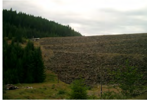
Figure 3-66 Smith Dam - July 22, 2006
