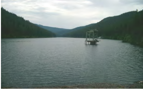
Figure 3-65 Smith Reservoir with inlet to penstock - July 22, 2006
