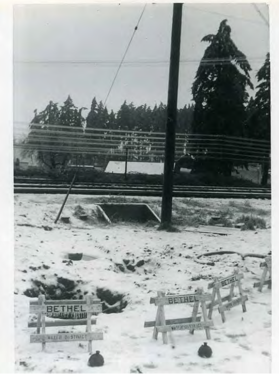
Figure 5-43 Bethel Water District job with safety signs
