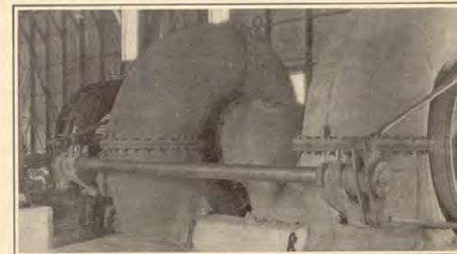
FRANCIS-FELTON TURBINES IN GENERATING STATION, EUGENE WATER-WORKS
