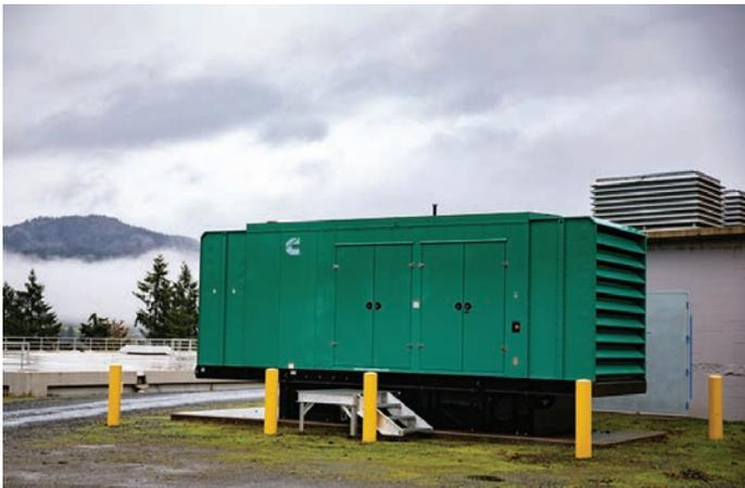
The backup generator at EWEB's Hayden Bridge Water Filtration Plant. The generator, one of several recent resiliency projects, made it possible for EWEB to maintain water service during the storm.
